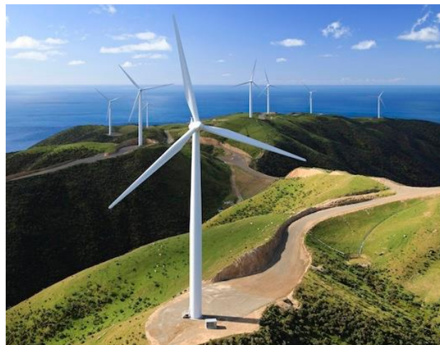
Figure 8: Horizontal axis turbines
