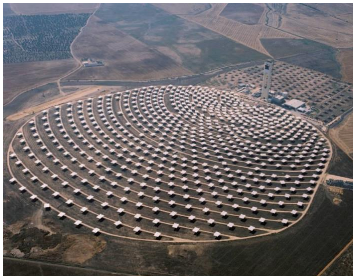
Figure 4: Thermodynamic solar power plant with flat mirrors and tower
